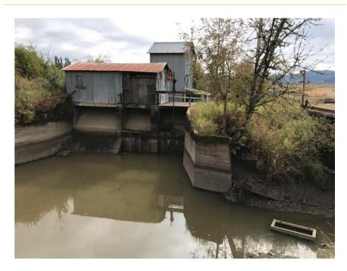
The new pumping station at **Wapato Lake NWR** is now up and operating as of February 23. The two new pumps have been consolidated into one new building on the dam structure that previously housed the non-operational 1930s era pump. The former operating pumps and
